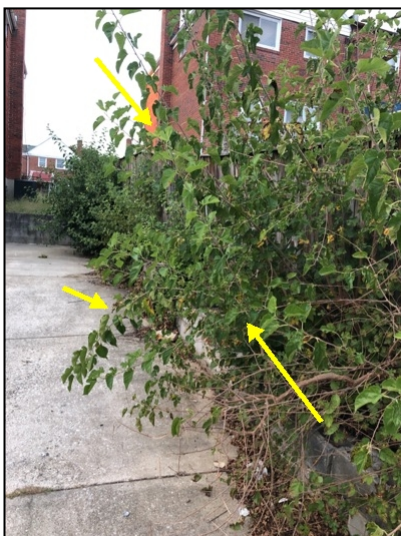
Heavy vegetation growth over driveway
