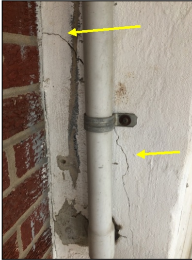
Cracked parging
