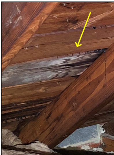
Area of previous leaking, dry during inspection
