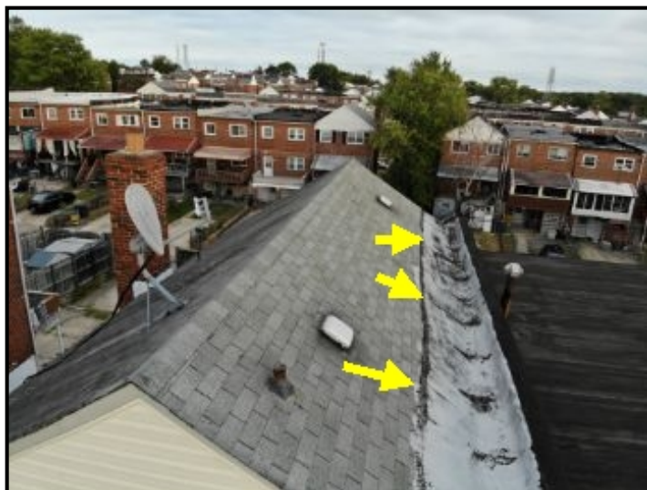
Roof Roof Condition
