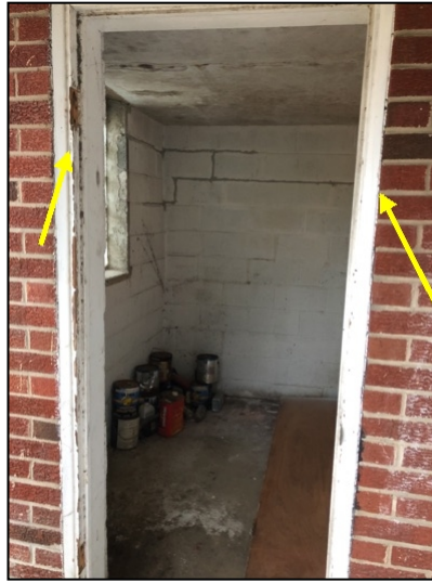
Door to storage area under deck dismantled
