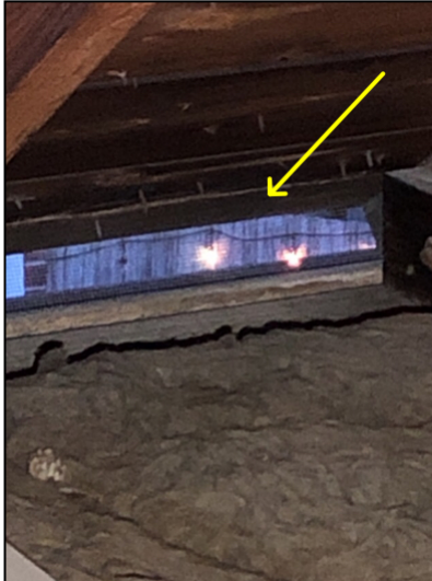
Soffit vents with screening installed
